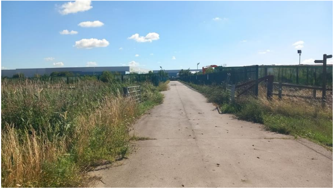
Figure 6-2: Condition of Access Road (Looking West)
