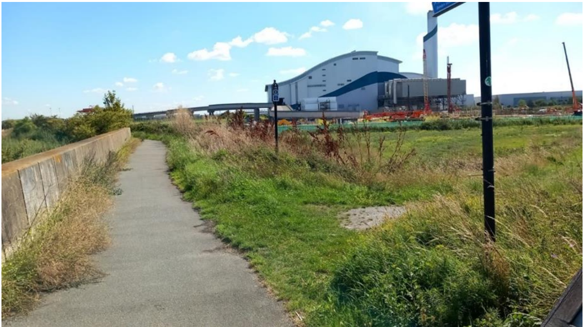
Figure 3-2: Condition of FP2 (Looking east at the junction with the England Coast Path (FP3/NCN1))
