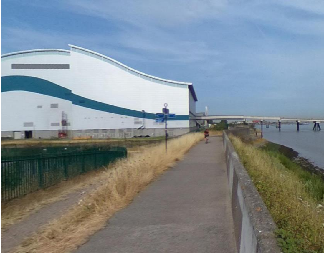
Figure 2-2: Condition of England Coast Path (FP3/NCN1) (Looking west at the Junction with FP4)
