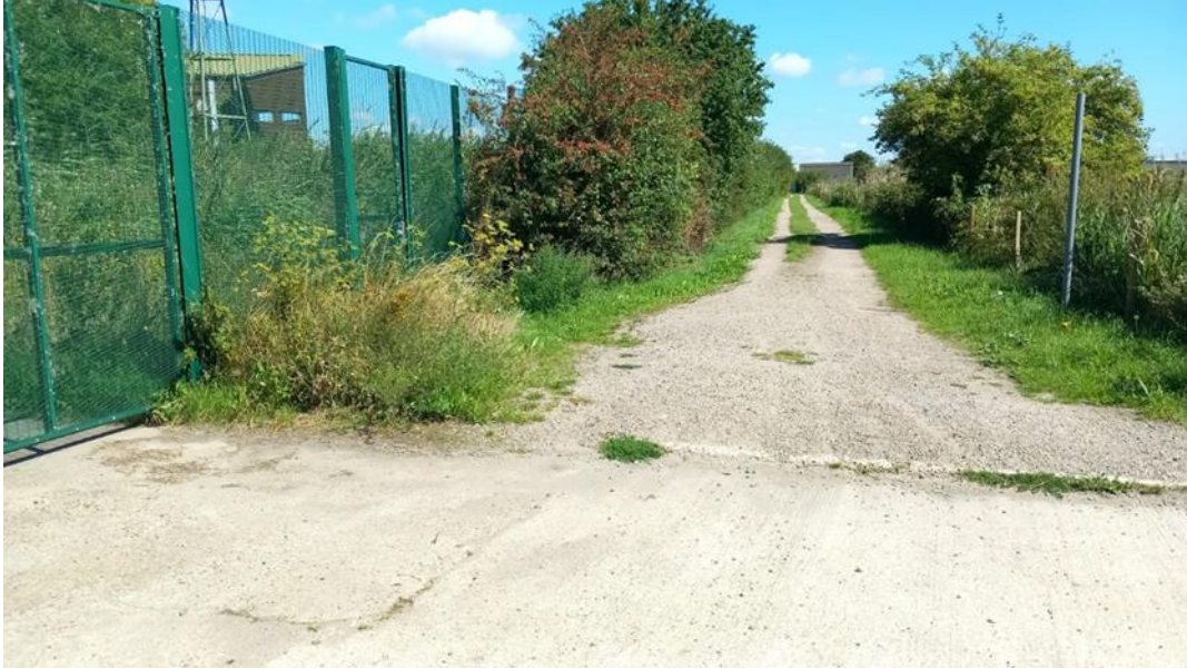
Figure 5-2: Condition of FP2 at Location 4 (Looking North East)
