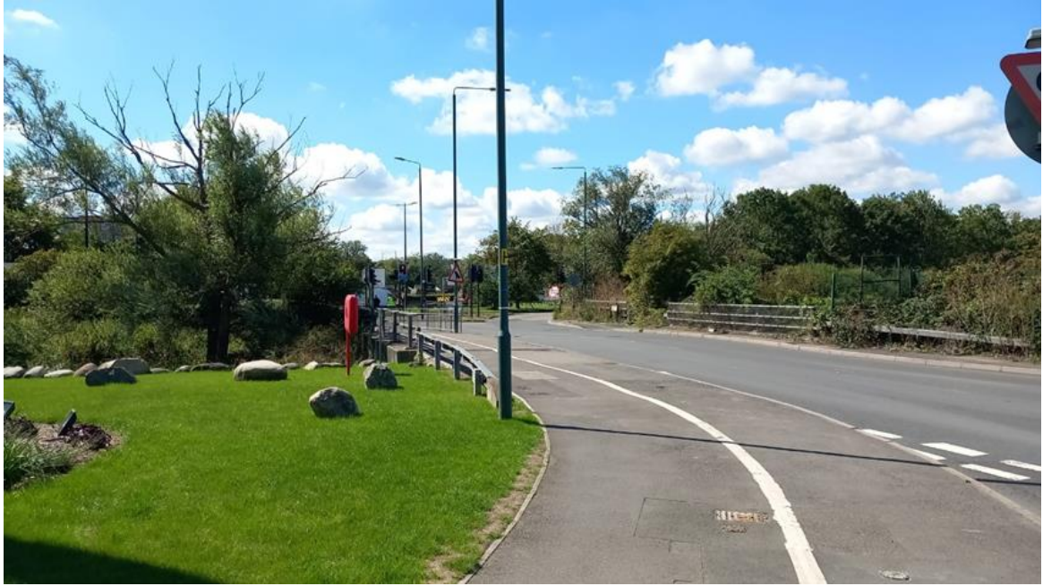
Figure 4-2: Condition of Norman Road (Looking south at the A2016)
