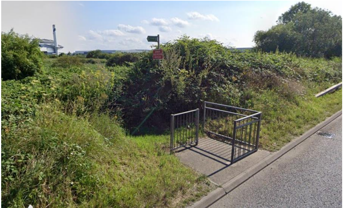
Figure 8-2: Condition of the Footpath North of Eastern Way (Looking North) 3
